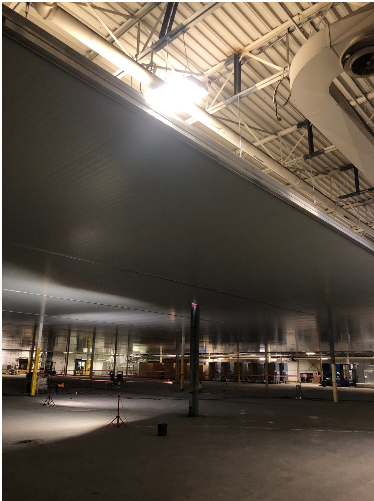
Figure 2: Dry Room Ceiling Plenum installed
