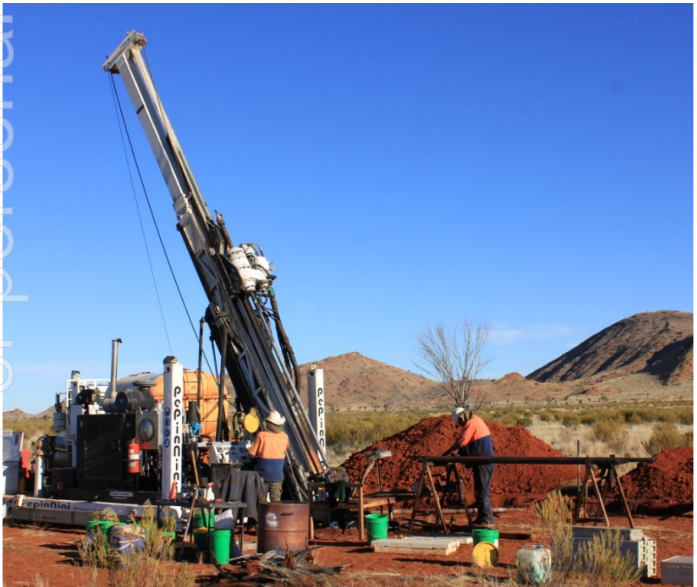
Photo 17 – PepinNini Diamond Core Drilling Rig
