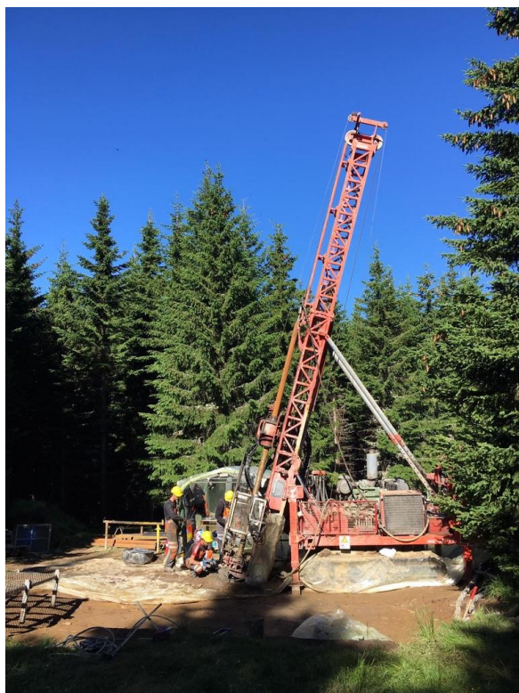
Figure 2: Drill Rig II - in operation
