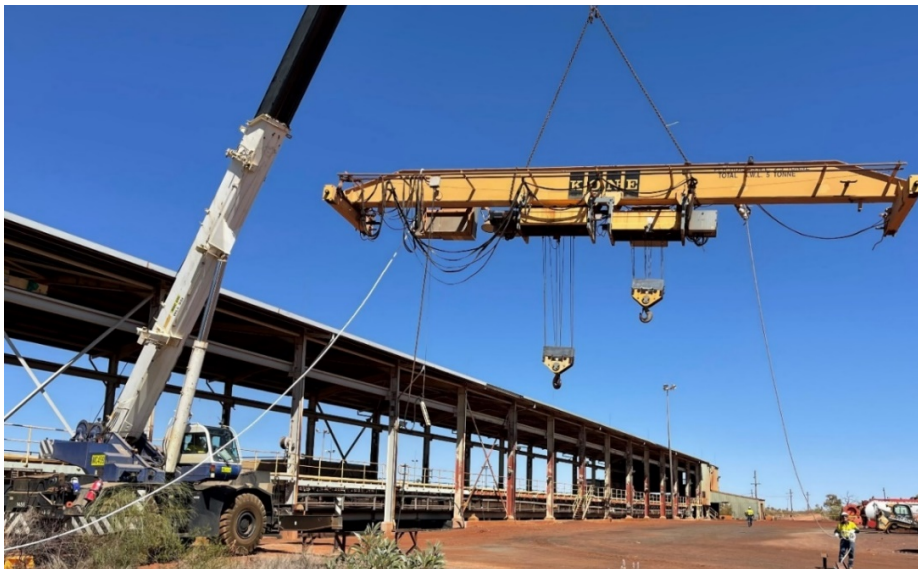
Image 1 / Overhead crane removal from Electrowinning Plant
