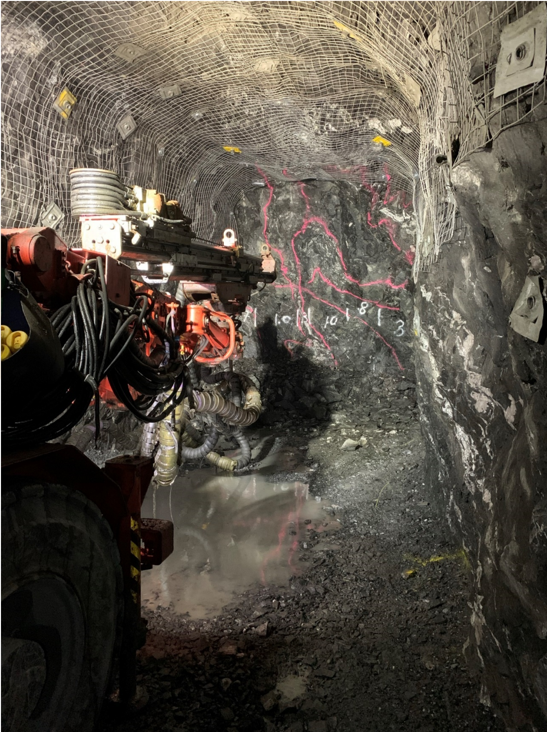
Ore drive underground at Golden Eagle
