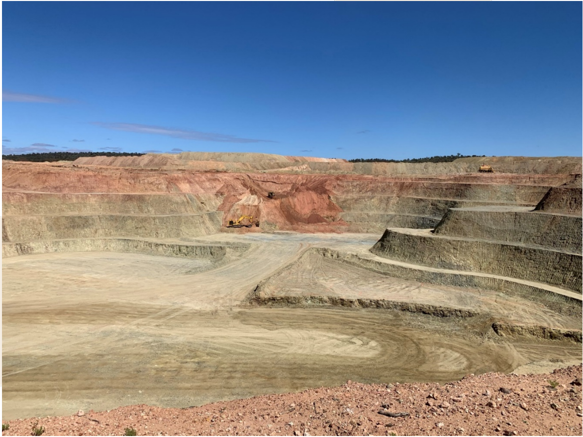
Riverina open pit (looking west) showing rehabilitation work of slip underway.
