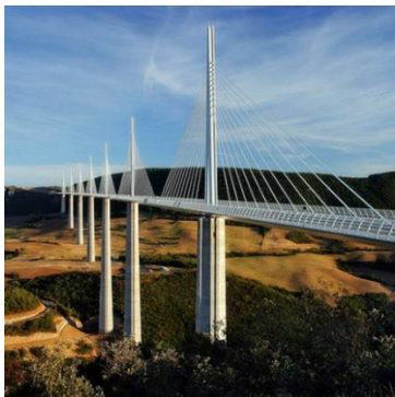
The Millau Viaduct in southern France was constructed using HSLA Steel containing 0.025% niobium; reducing the weight of steel and concrete by 60%
