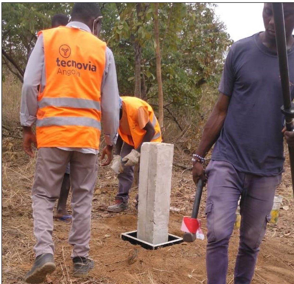
Figure 5 - Cabinda Phosphate Project, licence marker installation.
