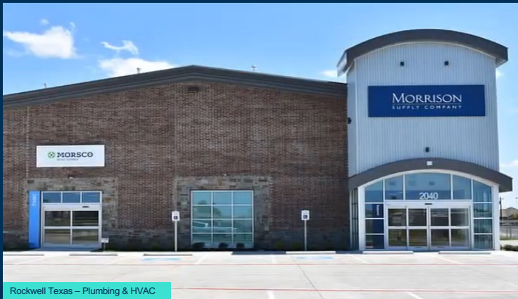
Rockwell Texas – Plumbing & HVAC
