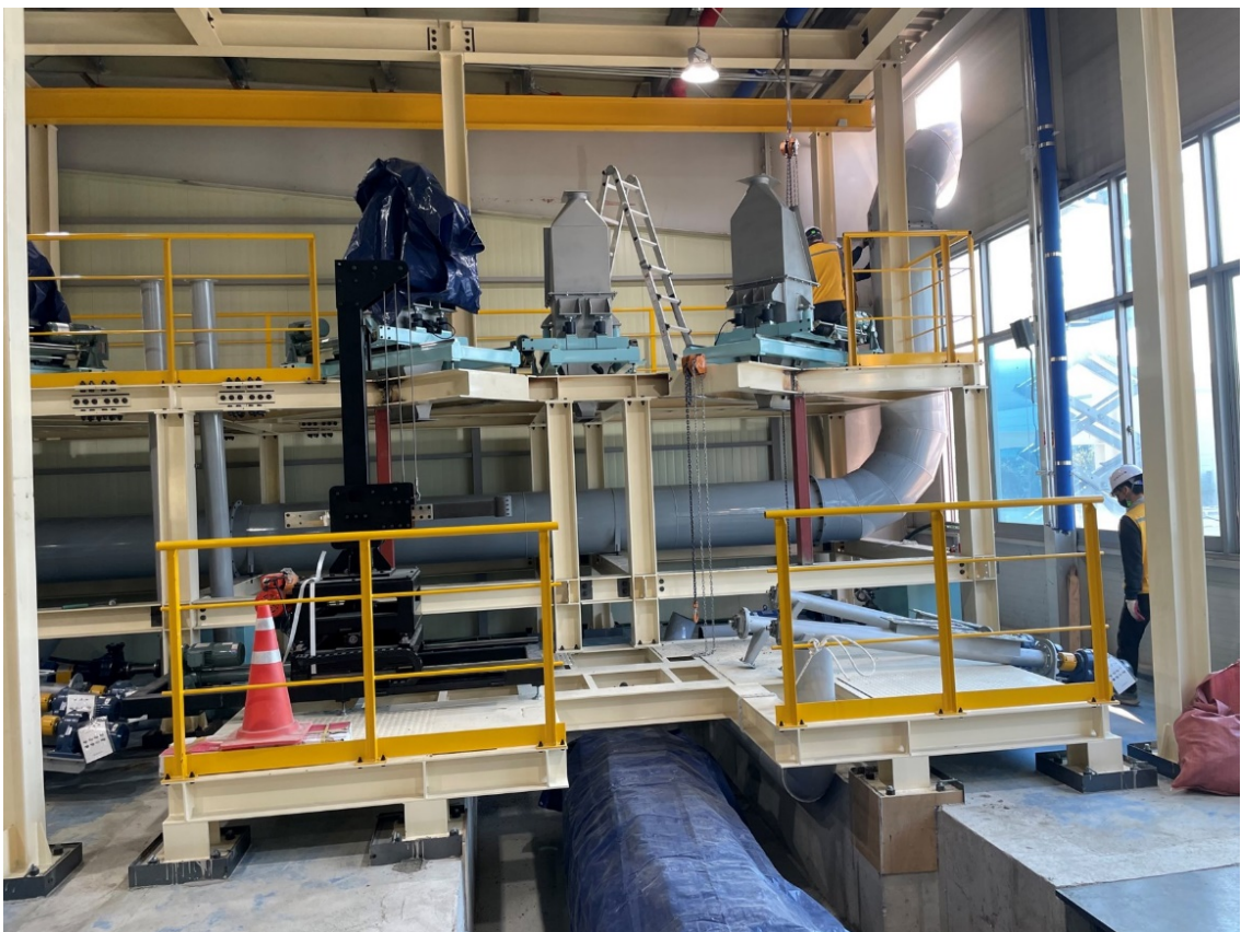
Figure 3 - Installation of Neodymium Furnace Infrastructure
