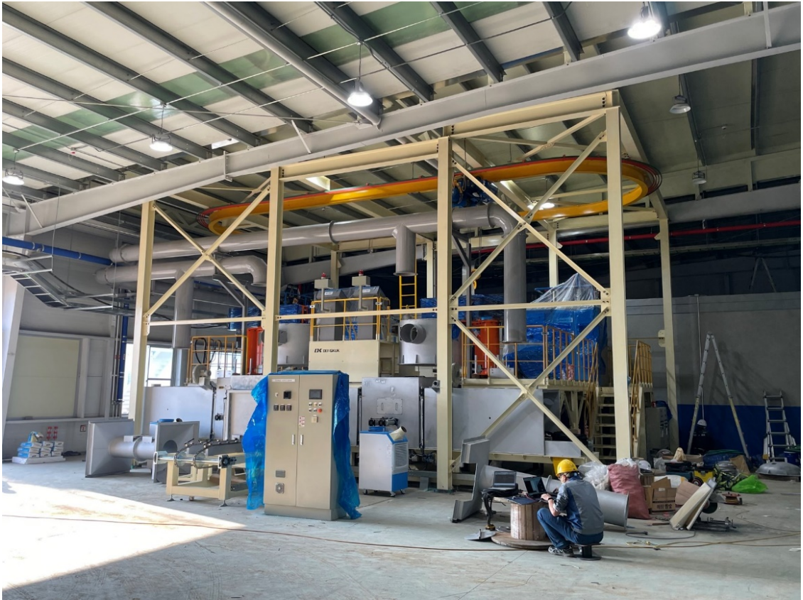
Figure 2 - First two Titanium Furnaces Installed
