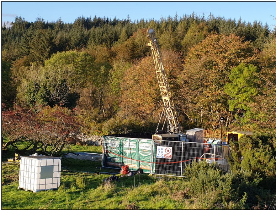
Figure 1: Photo of the drill rig set up on the first hole.
