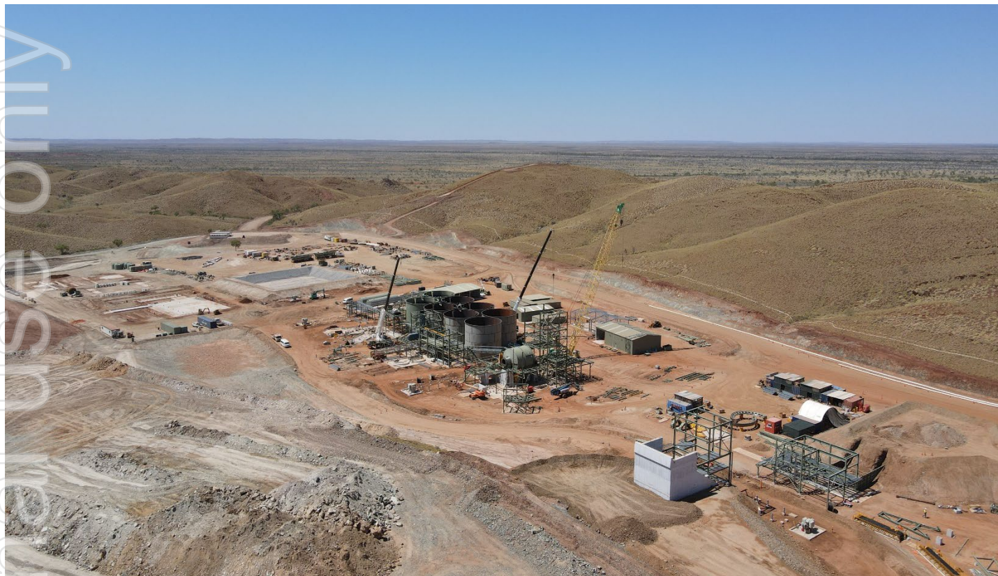
Figure 1: Overall Site View
