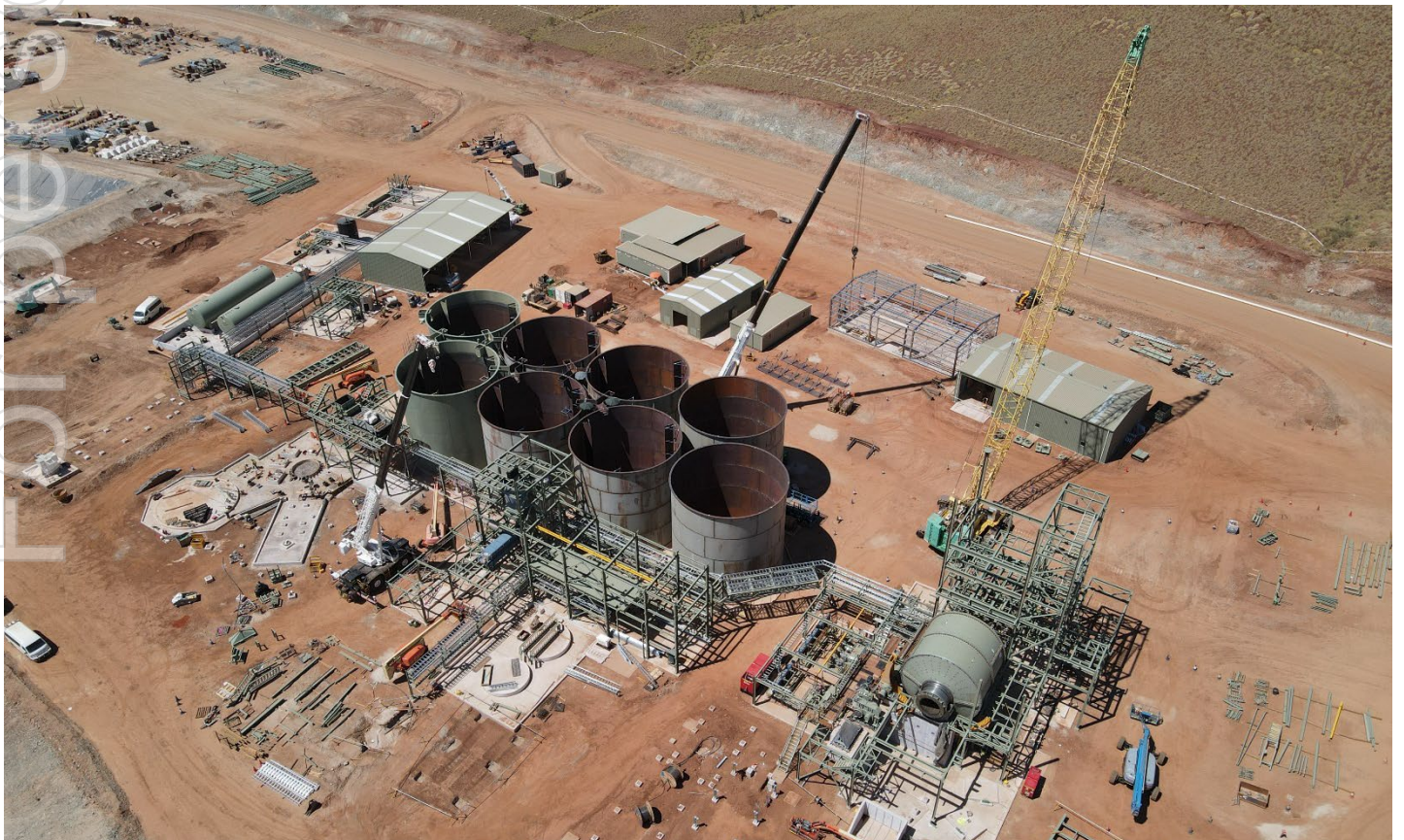
Figure 2: Mill and CIL tank area
