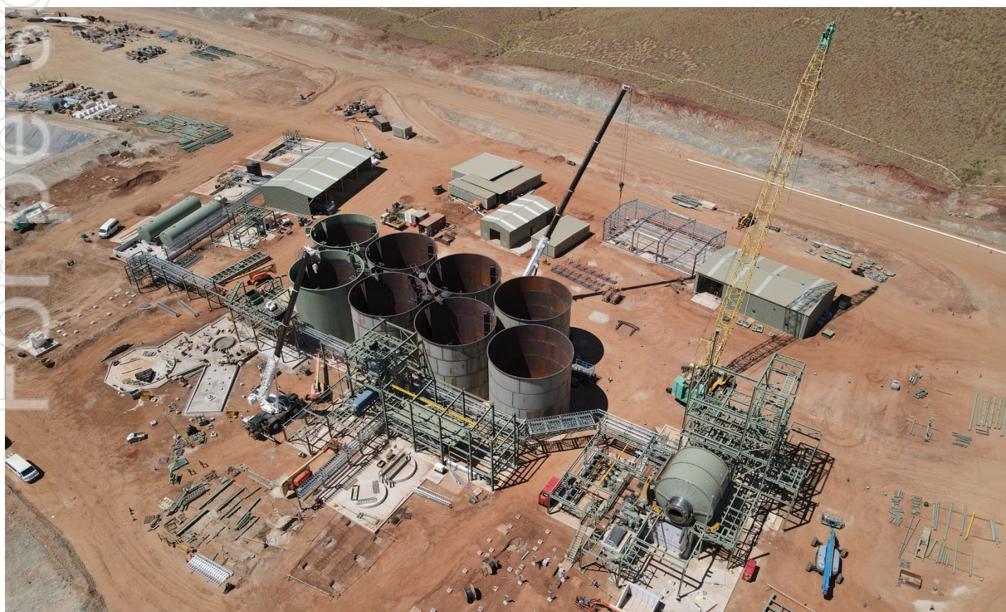
Figure 2: Mill and CIL tank area
