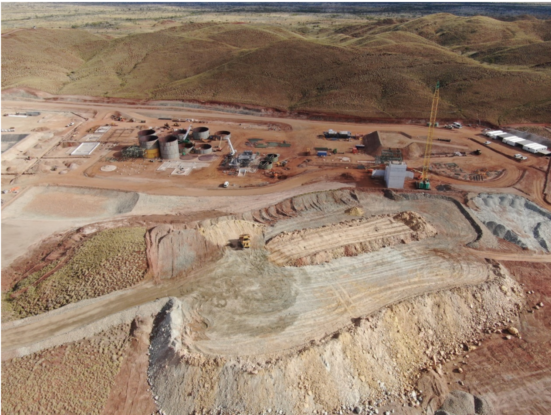
Figure 5: First ore on ROM Pad
