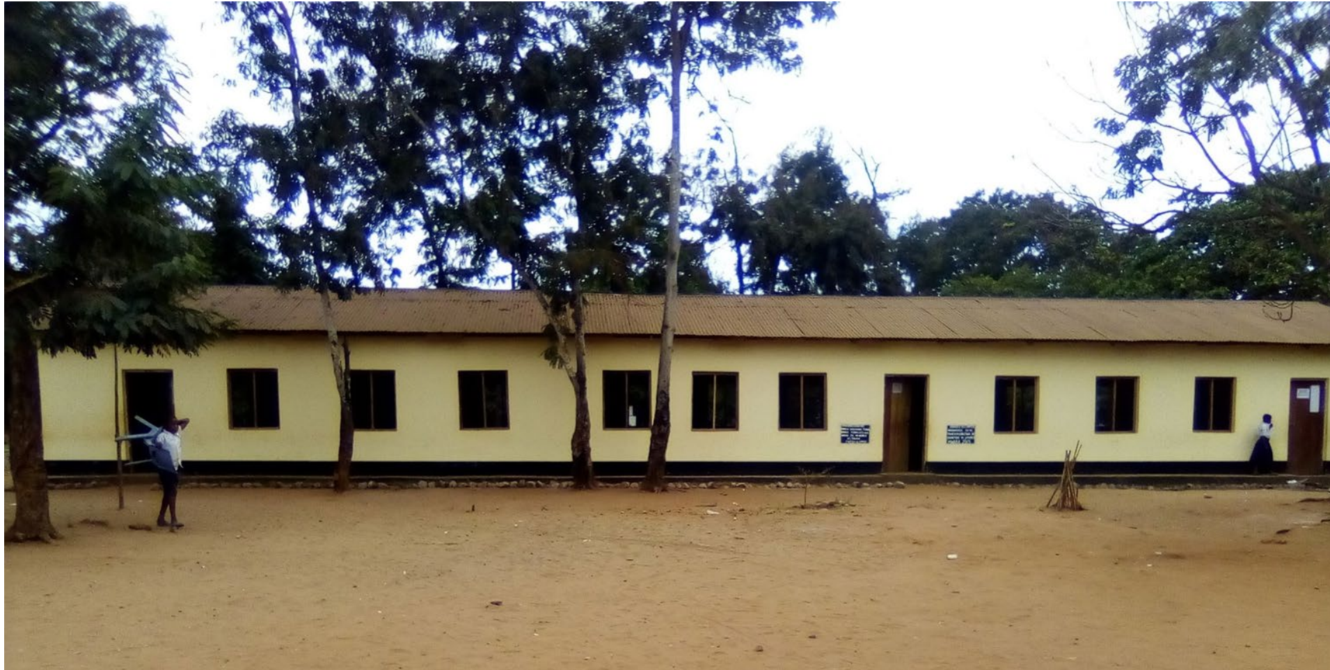
Figure 5. Renovated Classrooms At Matambarale Primary School
