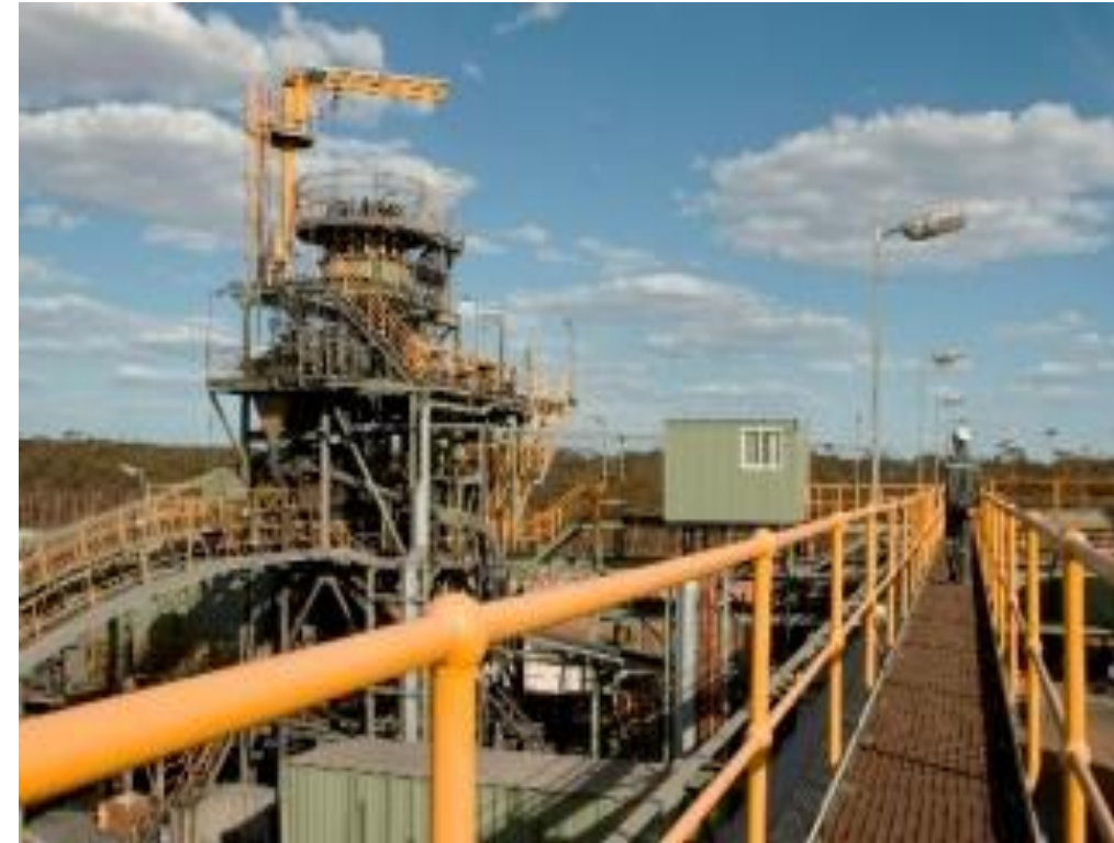
Lake Johnston processing plant
