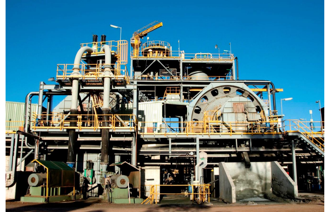
Black Swan 2.2Mtpa milling circuit Plans to refurbish and de-rate to 1.1Mtpa throughput
