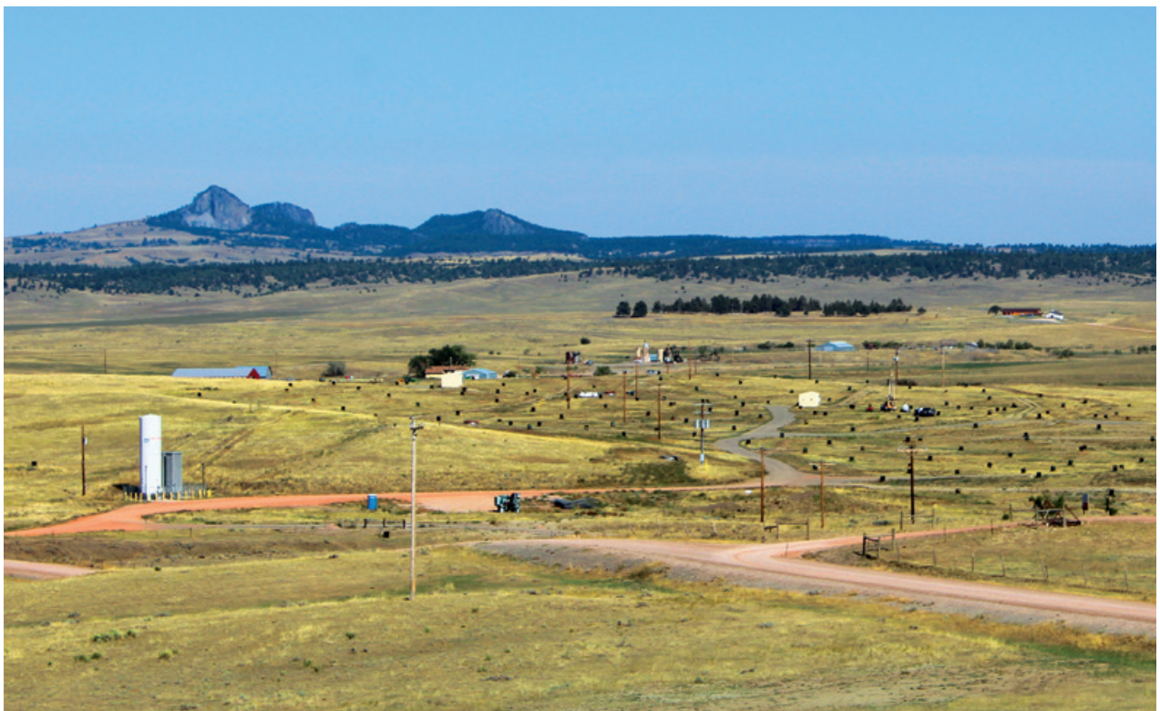
Figure 2: Lance Project, Wyoming, USA
