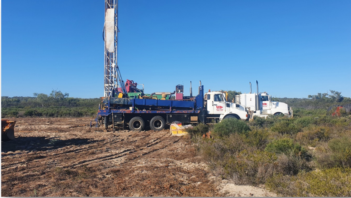
Figure 6 - Water Bore Rig onsite
