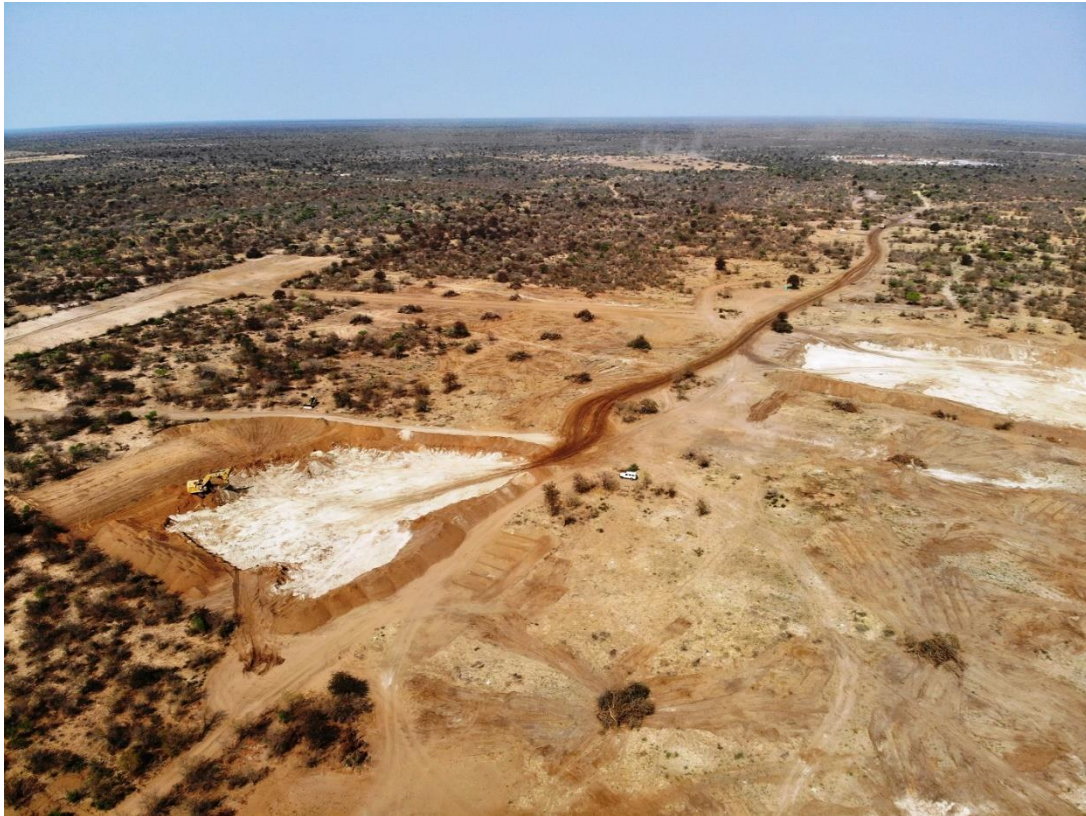
Figure 4: Clearing of topsoil T3 Stage 1 Open Pit and for the process plant and accommodation village in the background.
