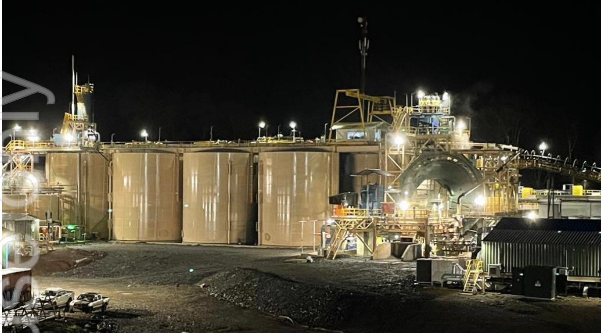
Figure 2 | Okvau Gold Mine Processing Plant
