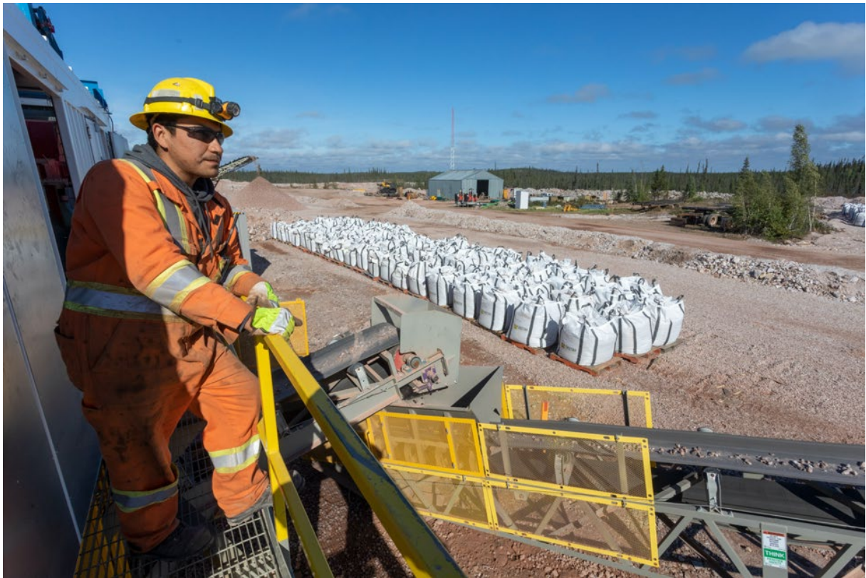
Product staging area at ore sorter reading for relocation to barge lay-down
