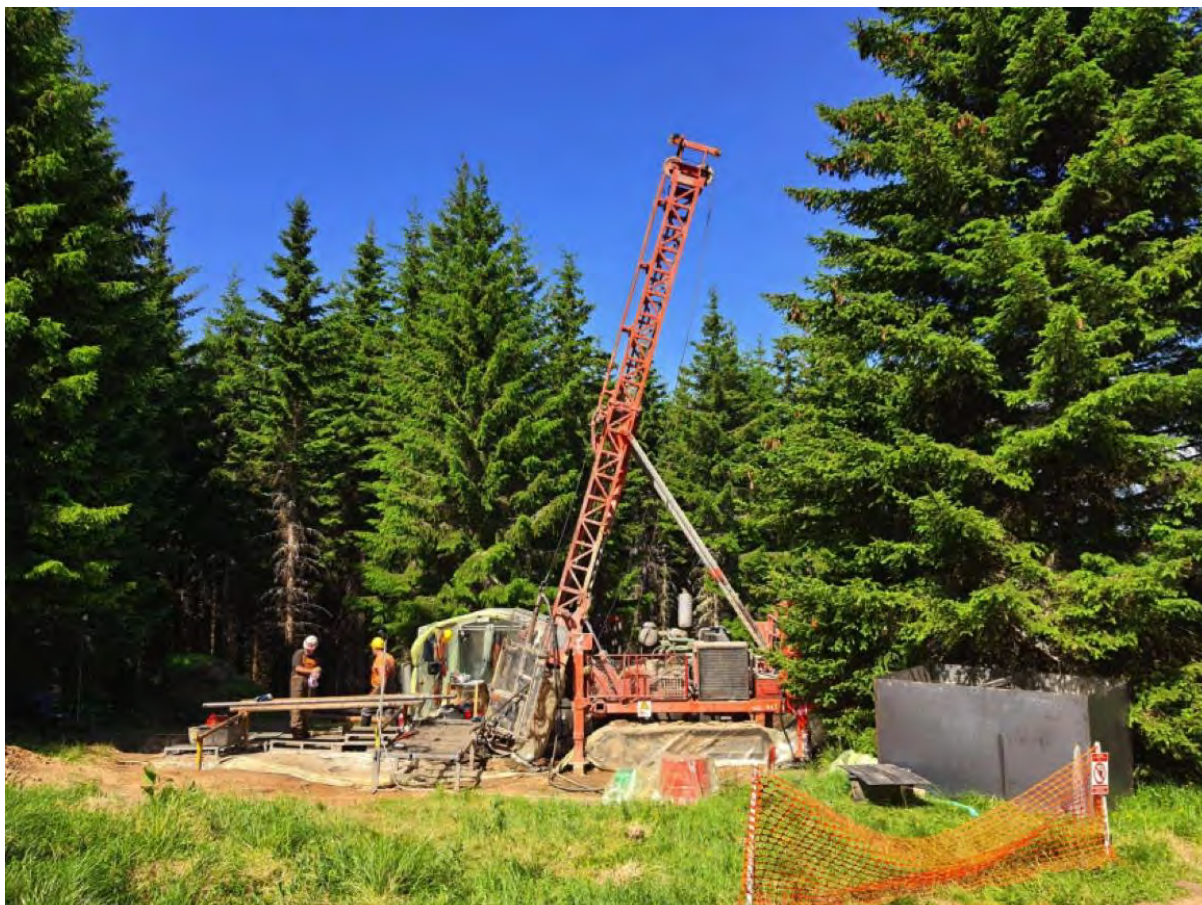
Figure 2: Drill Rig II - in operation
