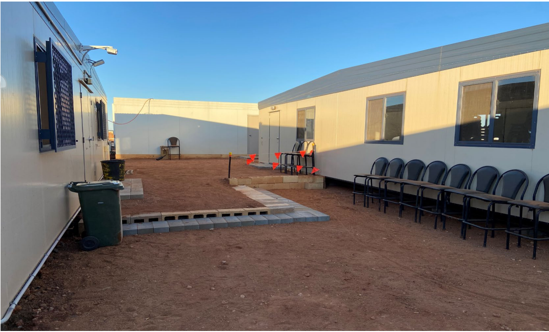
Figure 2: Operational fly camp
