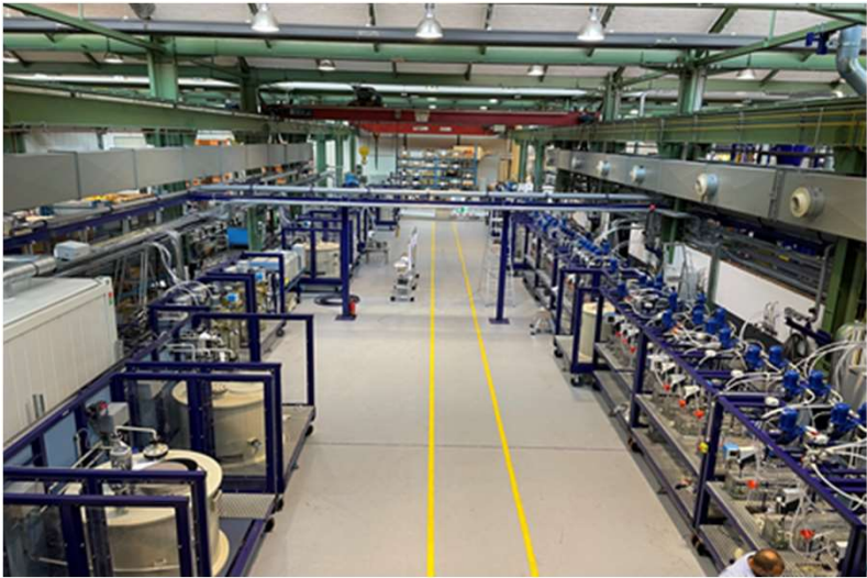
Dedicated facility at SMS Manufacturing Headquarters Hilchenbach, Germany
