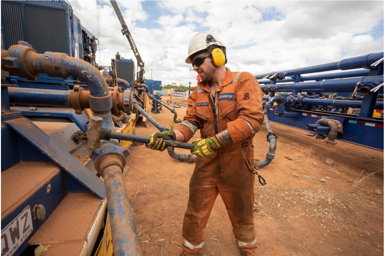
Above: Schlumberger field crew rigging up for Carpentaria-1 hydraulic fracture stimulation
