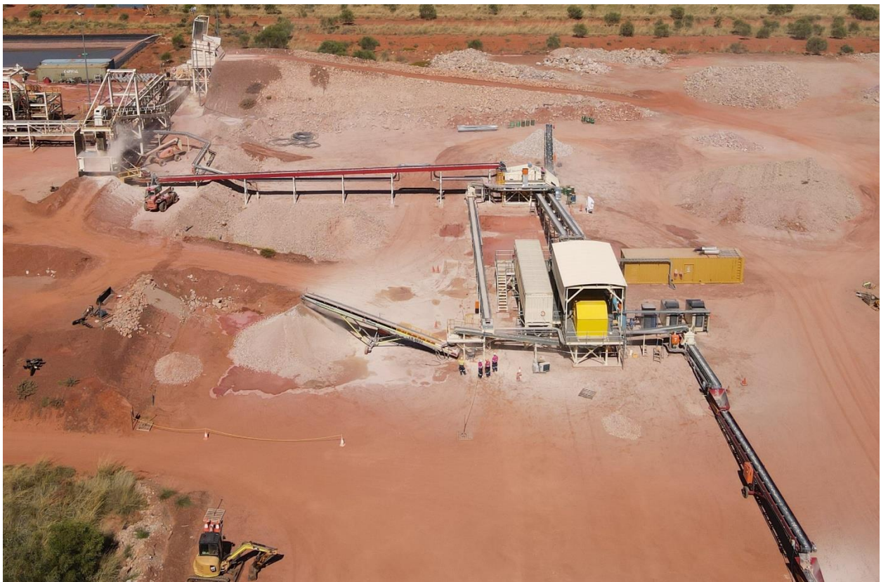
Figure 1: Operational ore sorter system
