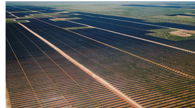
Prospero Solar Project, Texas
