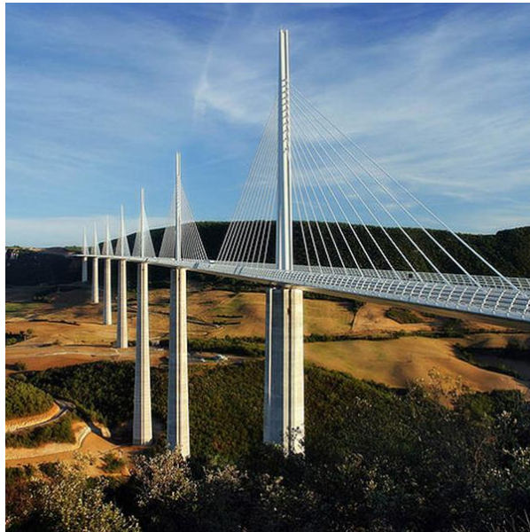
The Millau Viaduct in southern France was constructed using HSLA Steel containing 0.025% niobium; reducing the weight of steel and concrete by 60%
