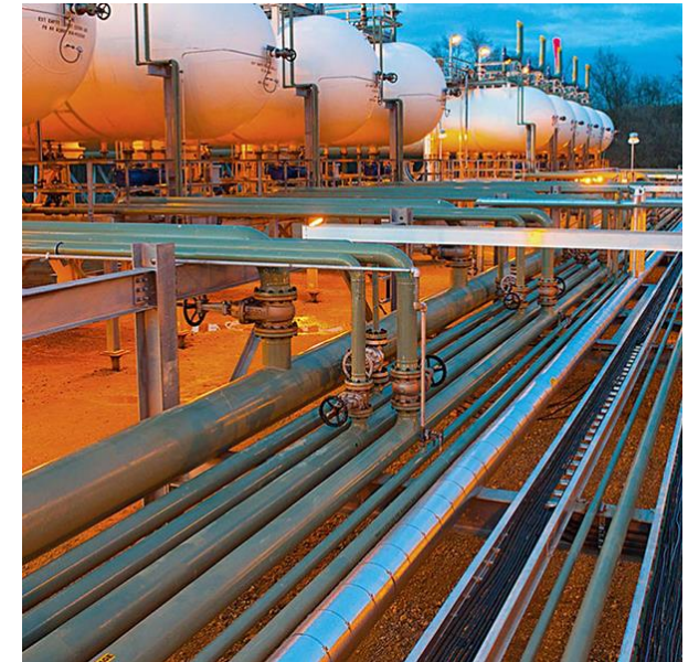
Most of the world's 3.5m kms of high pressure gas and oil pipelines contain niobium to make them safer, lighter and able to transport large volumes of hydrocarbons at higher pressures.
