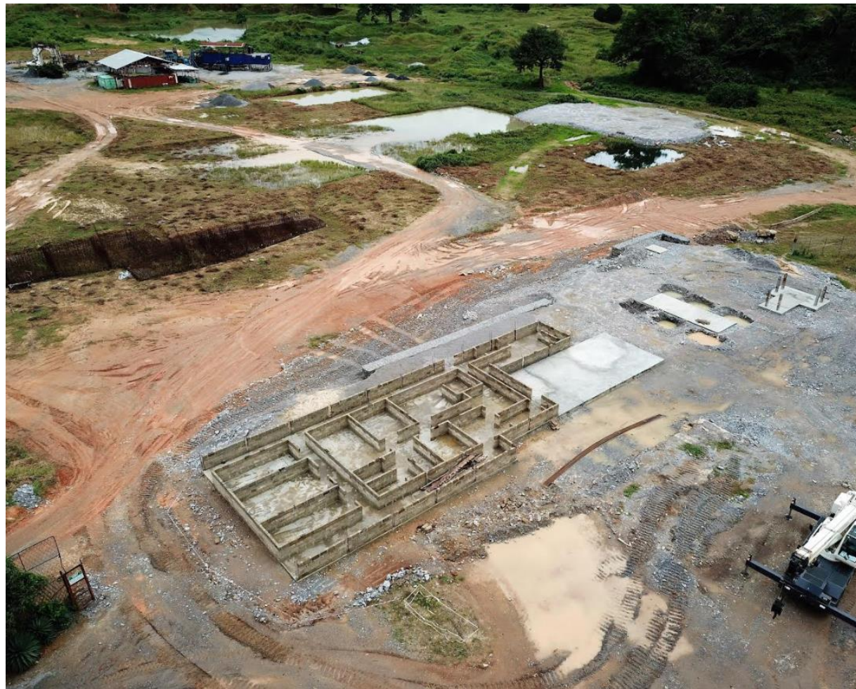
Foundations for 25tph plant, within close proximity to the current 5tph plant
