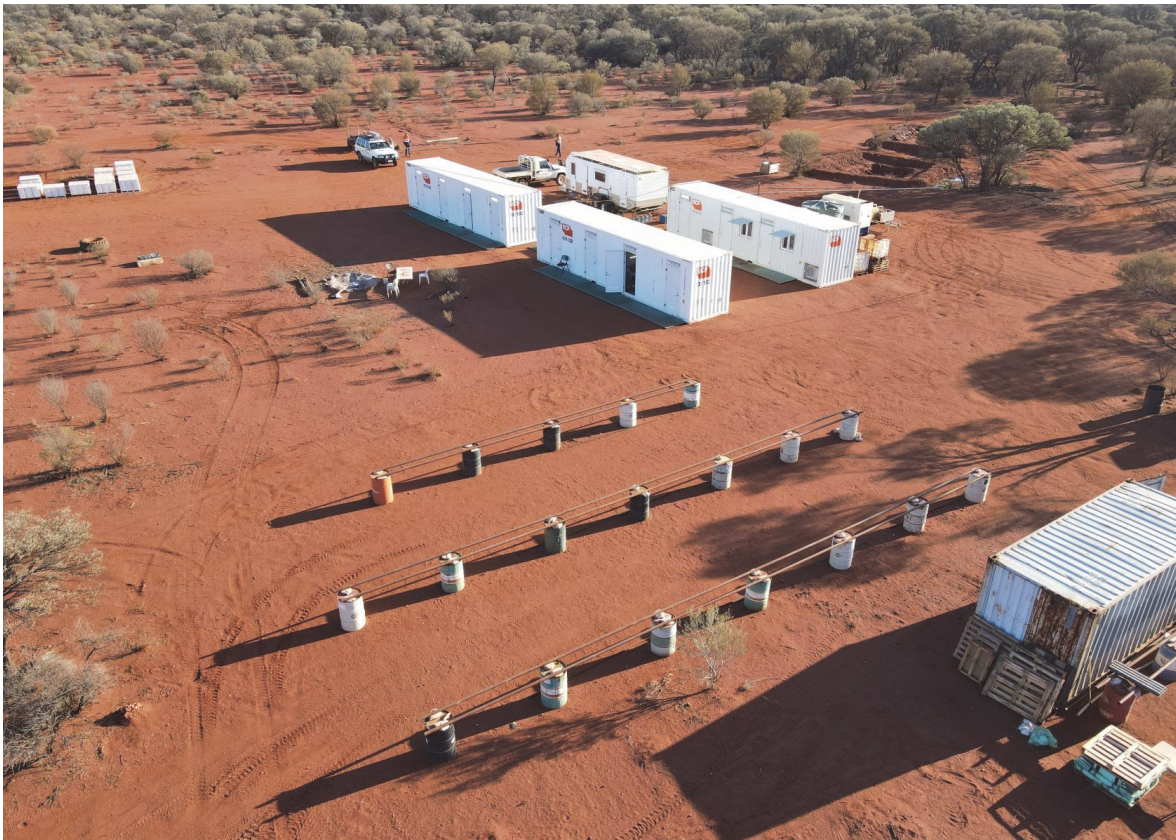
Above: aerial photo of the accommodation and work camp at Mt Alexander
