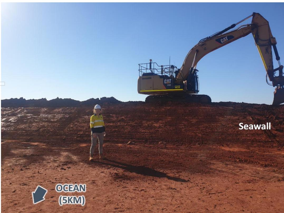
At the southern trial pond, seawalls will be constructed on three sides with an internal levee separating the trial pond (future Pond 0) from future Pond 1 (refer Figure 4). Geofabric will span the 20m width of the embankment bases to provide stability for the three-metre-high clay layer walls which will be protected from the ocean currents by rock armour. The southern trial pond will incorporate construction methodology, materials and equipment learnings from the northern embankment trial.
