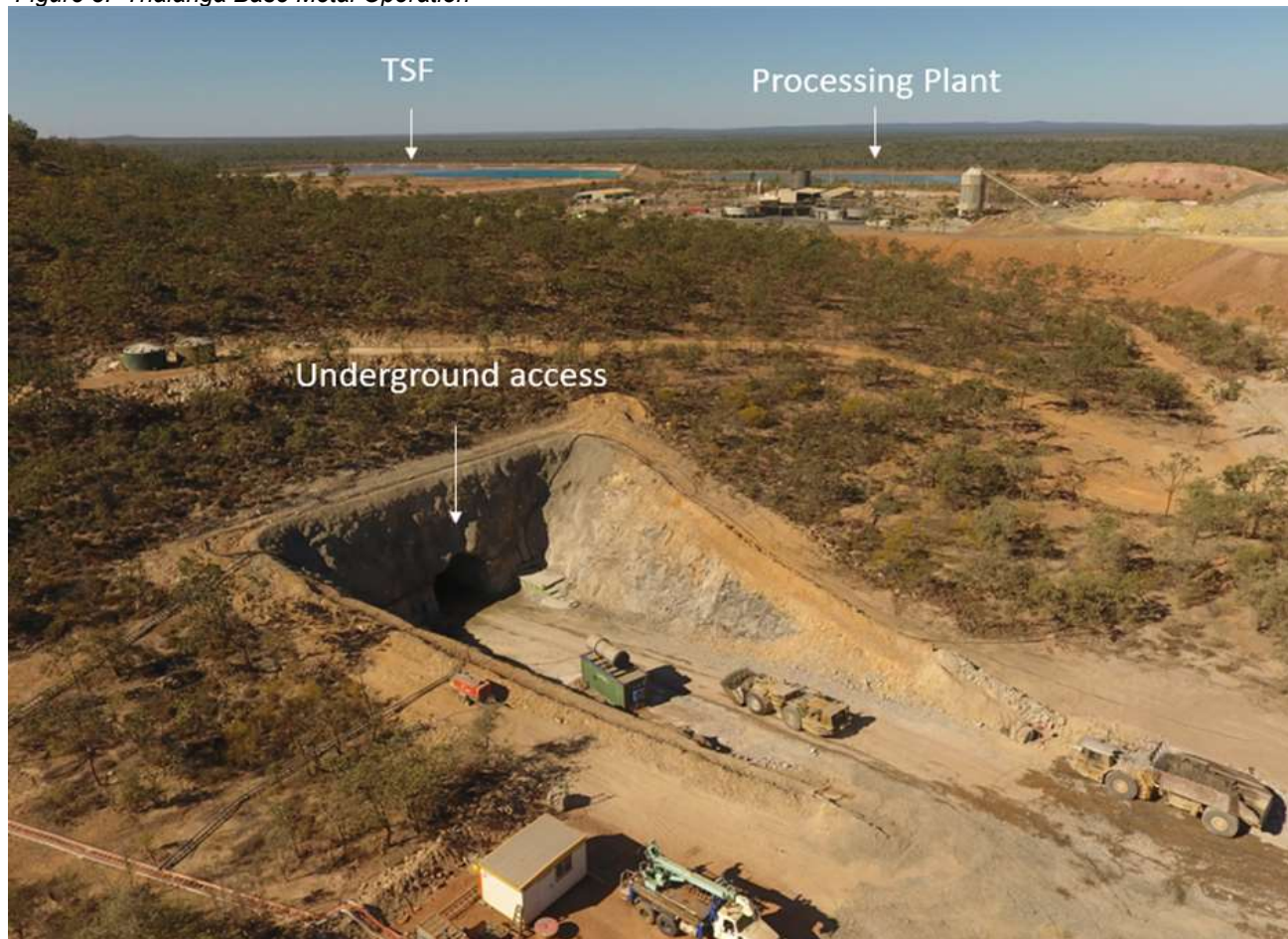
Figure 3. Thalanga Base Metal Operation
