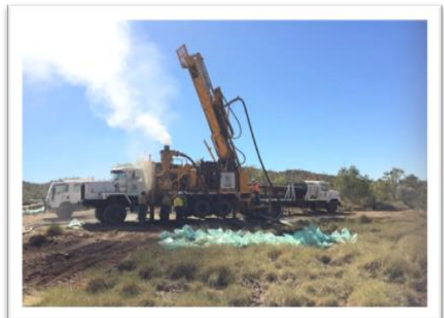
Image 2. RC Drilling of Hole TR17RC07
