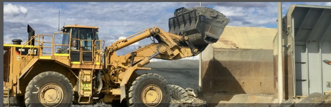
First bucket of Kundana ore into the Mungari crusher - 18 Aug 2021
