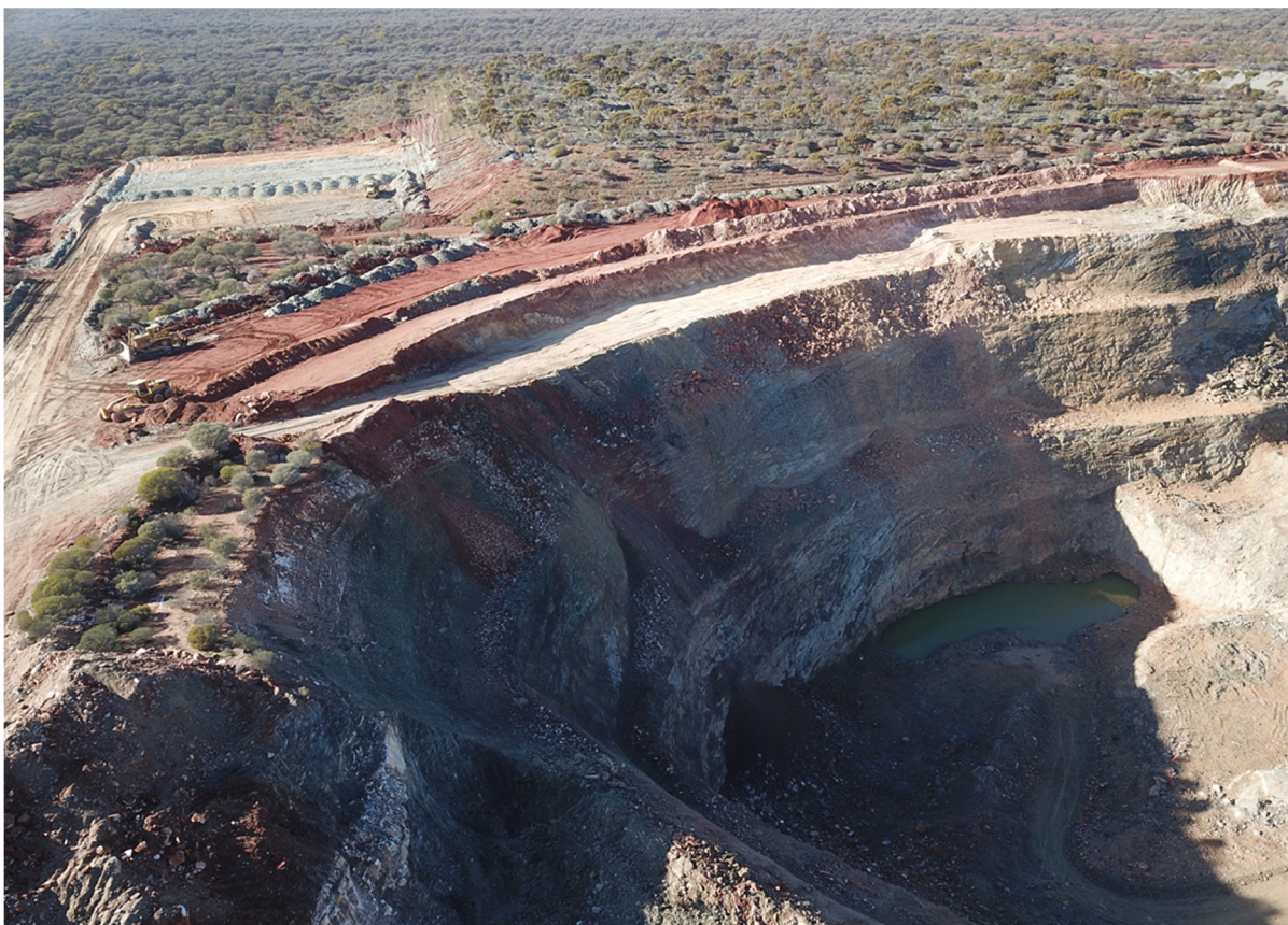
Plate 2 Granny Venn Cutback, bench development and Haul Road Construction
