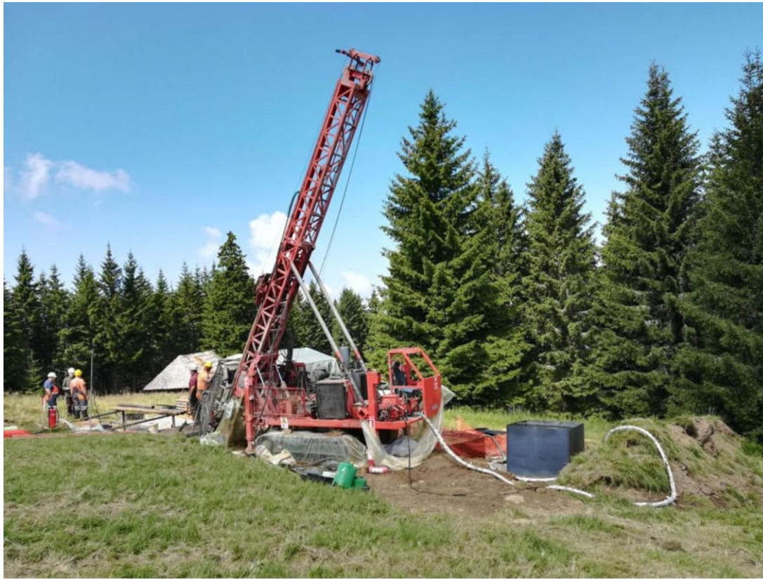
Picture 1: Drill rig B operating at P18-20
