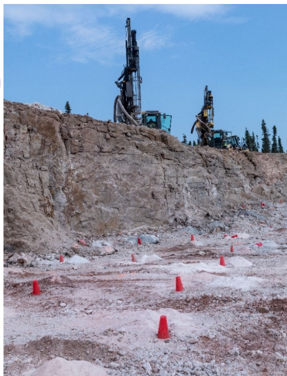
Drilling to expand Nechalacho pit
