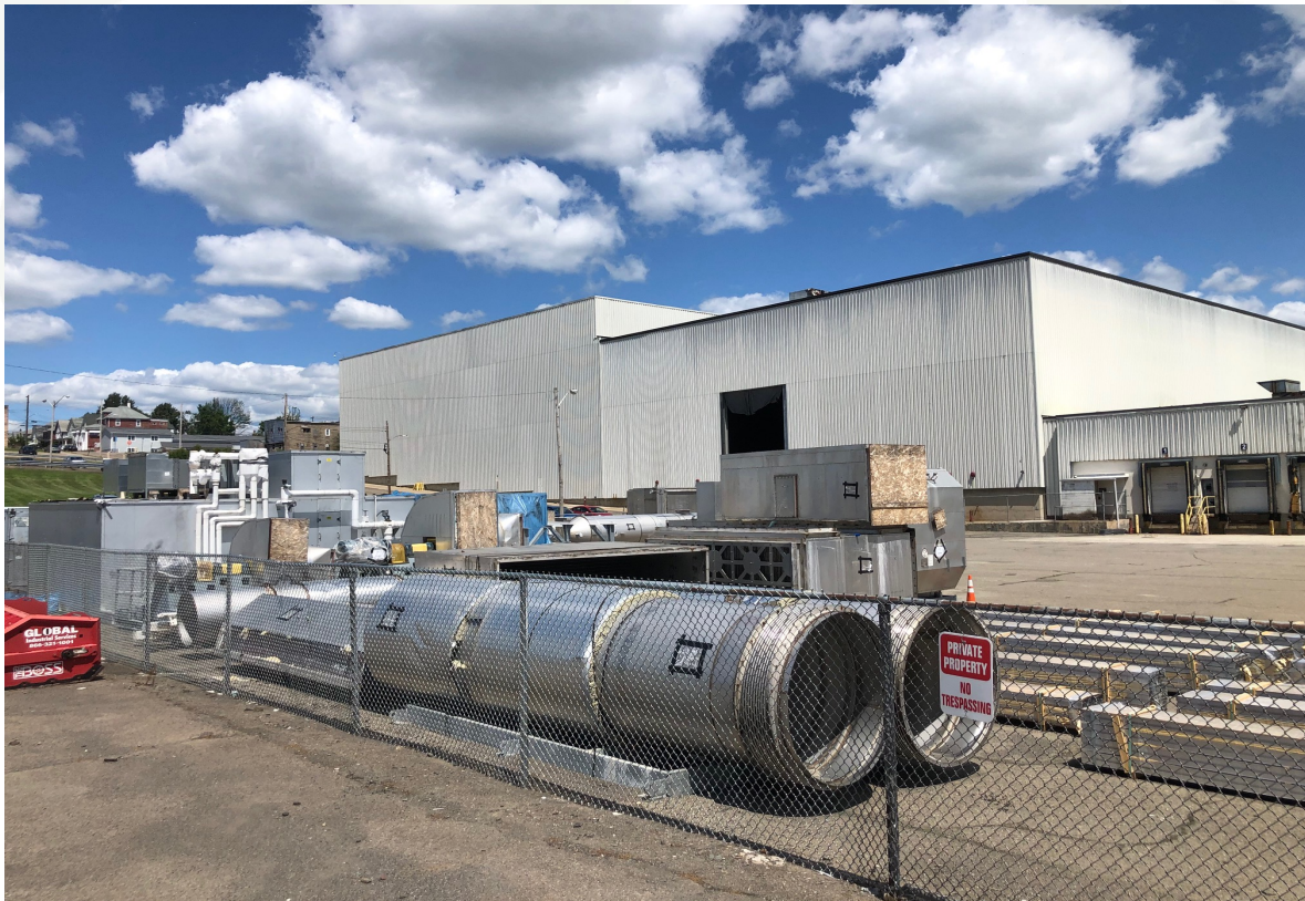
Figure 4: External Condenser Systems moved to final location
