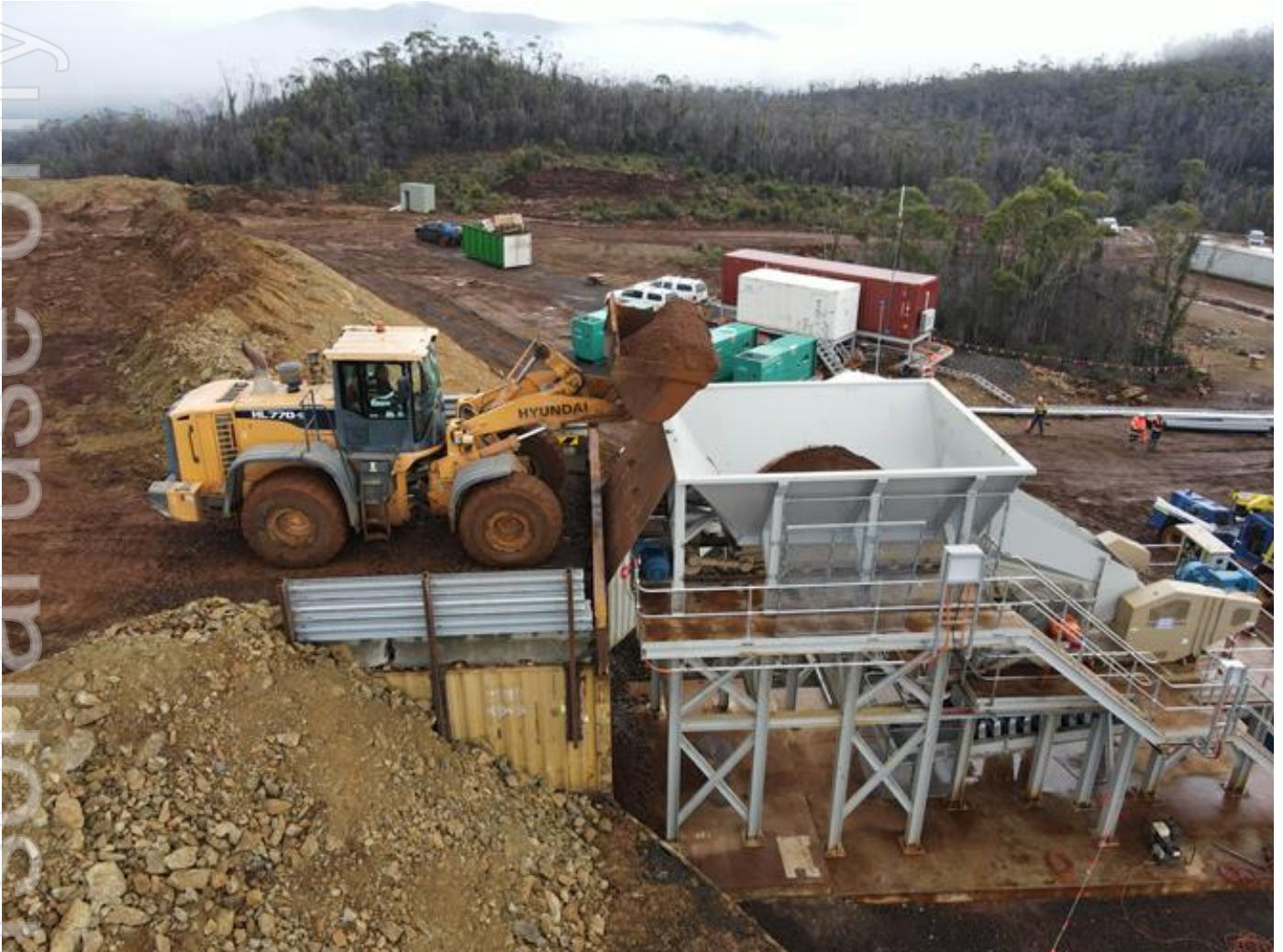
Figure 2 | Riley Wet Screening Plant as of 1st June 2021
