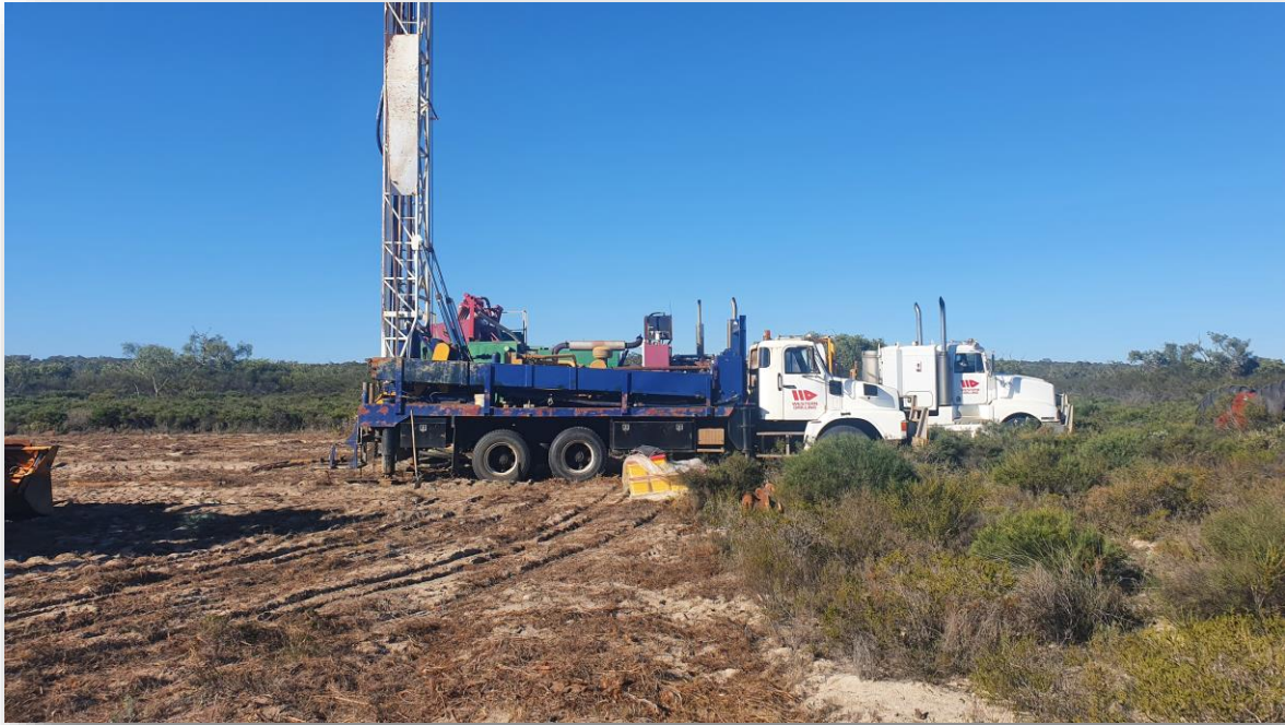
Figure 2: Water Bore Rig onsite
