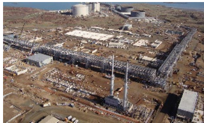
PLUTO LNG PROJECT - TEMPORARY FACILITIES WA Woodside Energy, $82m Dec 2008 – Dec 2012
