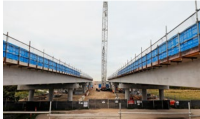
MORDIALLOC BYPASS PROJECT Melbourne, VIC MRPV, $375m 40% Decmil JV Oct 2019 – Current
