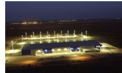
PORT HEDLAND WAREHOUSE HUB WA BHP, $32m Mar 2016 – Aug 2017
