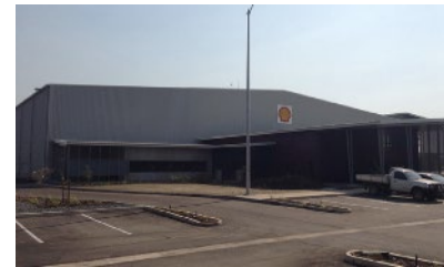
PRELUDE FLNG FACILITY DARWIN ONSHORE NT Shell Australia, $29m Mar 2013 – Jun 2014
