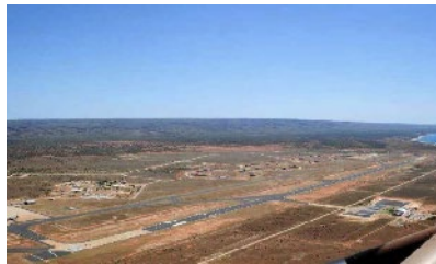
RAAF BASE LEARMONTH FUEL INFRASTRUCTURE WA Australian Defence Force, $19m Apr 2015 – Nov 2016
