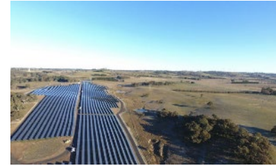
GULLEN RANGE SOLAR FARM NSW Gullen Solar, $20m Dec 2016 – Feb 2018
