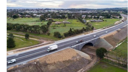
DRYSDALE BYPASS Drysdale, VIC MRPV, $92m June 2018 – June 2020
