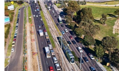
PLENTY ROAD DUPLICATION STAGE 2 Mill Park, VIC MRPV, $105m Jun 2019 – Current
