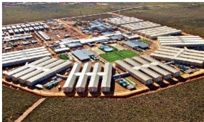
GORGON CONSTRUCTION VILLAGE (TDKJV) WA Gorgon Australia, $862m - 33% Decmil JV Jun 2009 – Jun 2013
