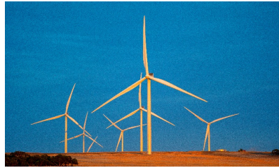
WARRADARGE WIND FARM WA Vestas, $72m Mar 2019 – Sep 2020
