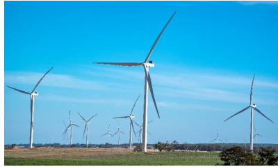
YANDIN WIND FARM WA Vestas, $80m Apr 2019 – Sep 2020
