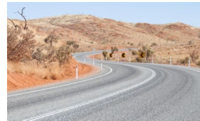
MOUNT WEBBER ROADWORKS Marble Bar, WA Atlas Iron, $71m Jan 2014 – Aug 2014
