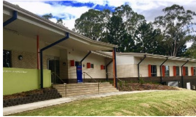
BONALBO MULTI-PURPOSE SERVICE MAIN WORKS Bonalbo, NSW NSW Health Infrastructure, $12m Dec 2016 – May 2018
