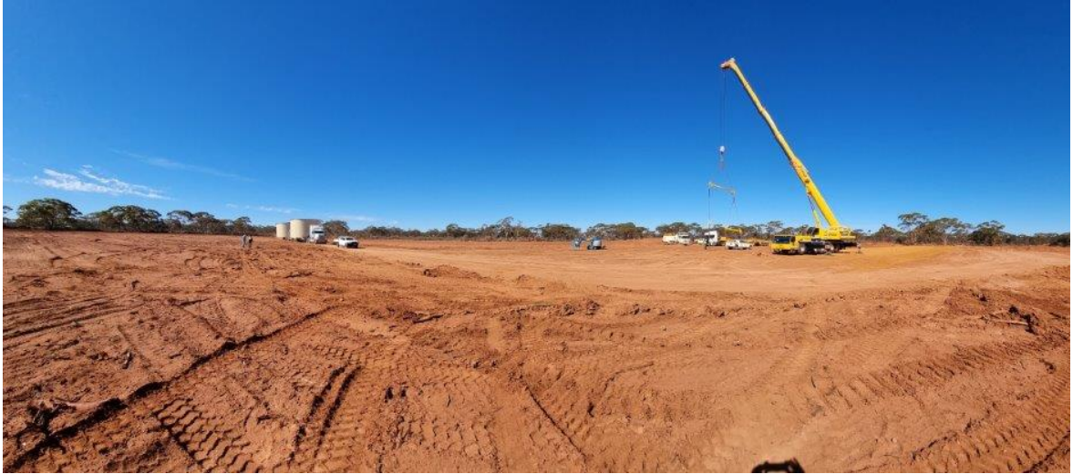
Preliminary Site works and delivery of tanks
