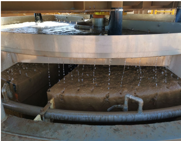
Commissioning of 2 nd Stack Cell
