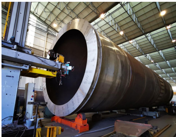
All 5 sections of kiln shell completed/close to completion
