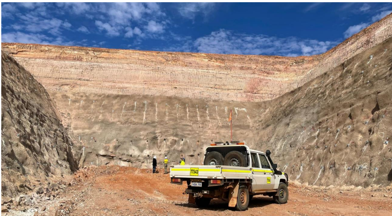
Figure 1. Box-cut with ground support works.
