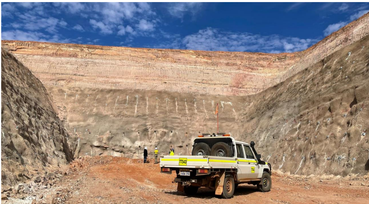
Figure 1. Box-cut with ground support works.
