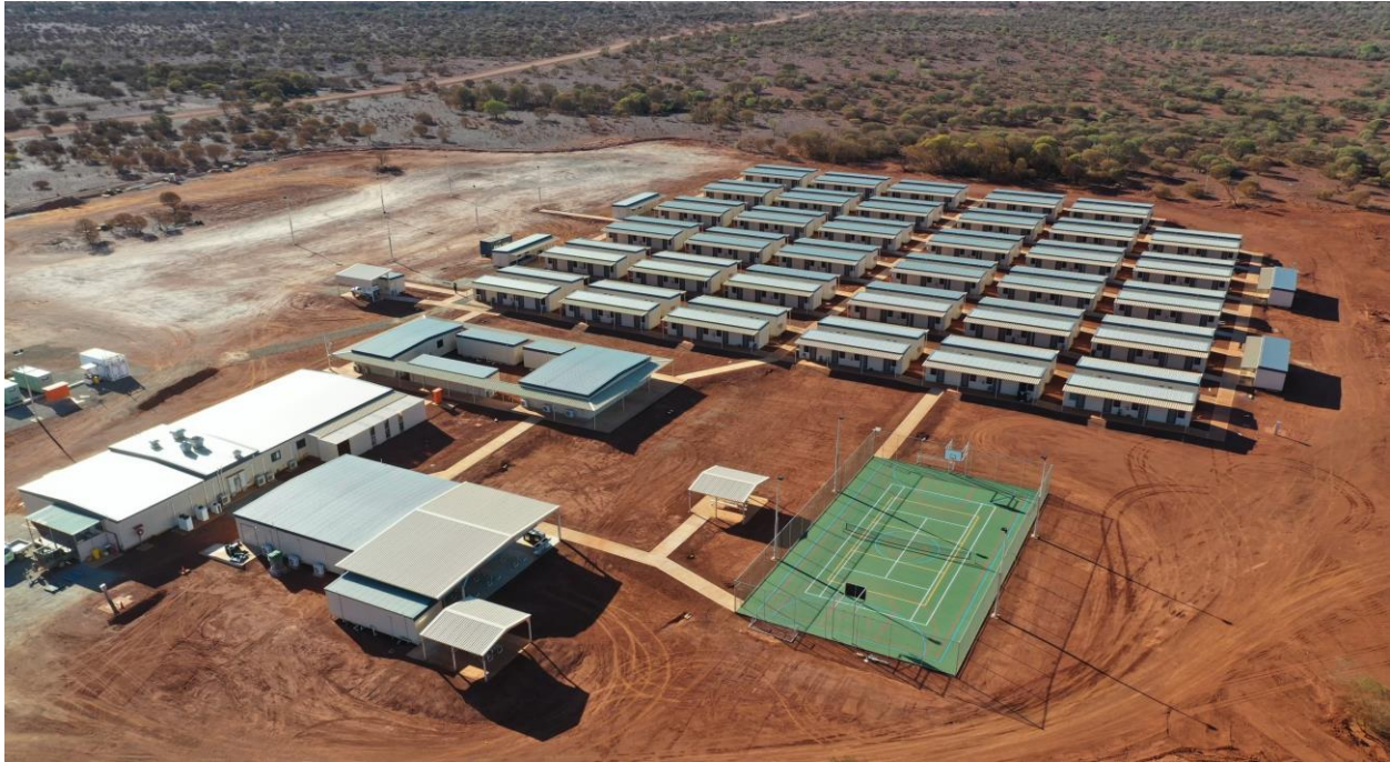
Figure 2. Completed 280 room Abra accommodation village.
