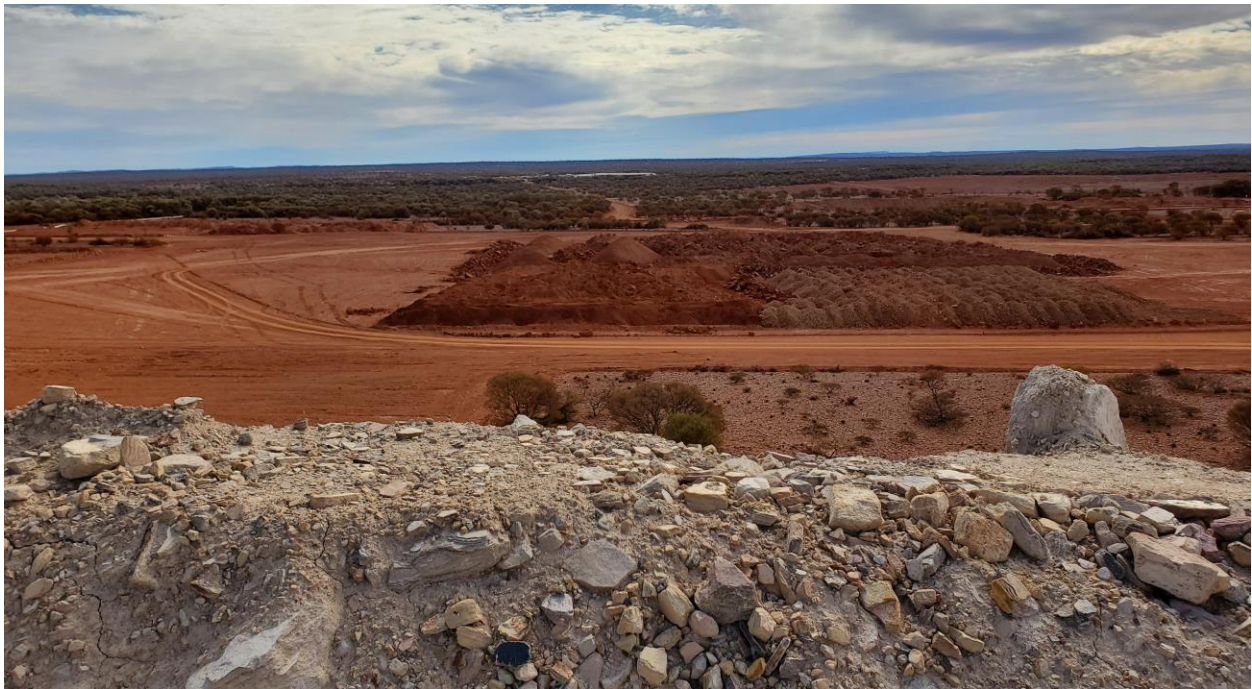
Figure 3. Cleared site of Abra's future processing plant (picture taken from the top of the ROM pad).
