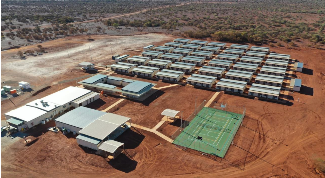
Figure 2. Completed 280 room Abra accommodation village.
