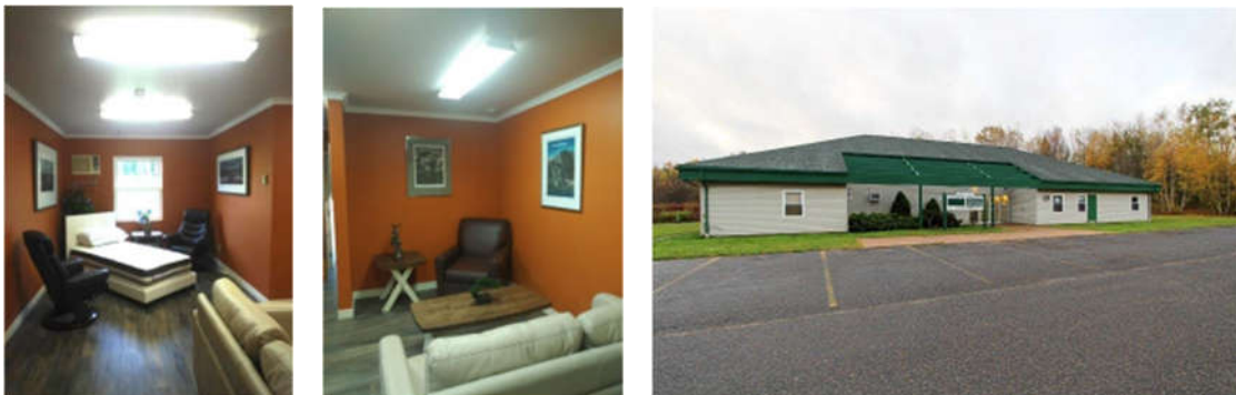
Images: Established 16,000 sq ft treatment facilities in Nova Scotia, Canada
