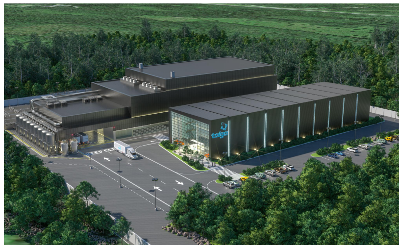
Luleå Anode Refinery
