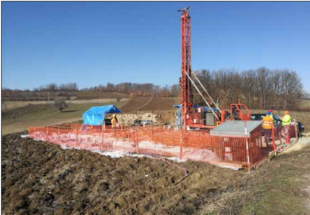
Figure 8-16: Drill rig at REK001 site in February 2020
