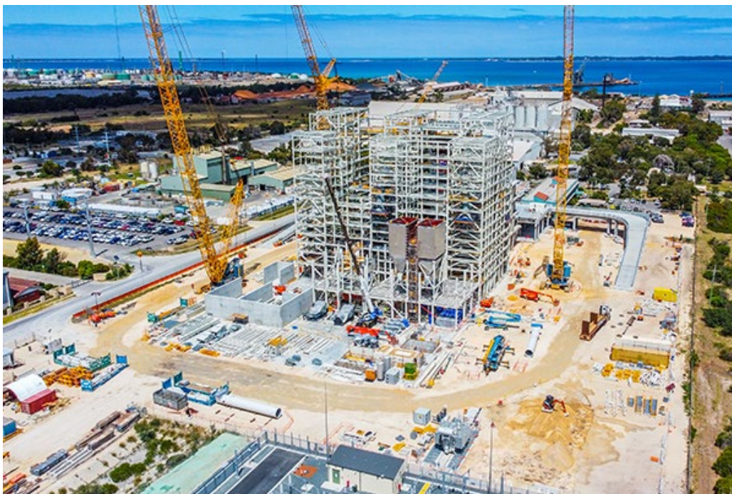
Image – Kwinana energy from waste construction site.
