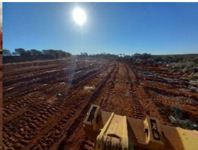
Haul Road Upgrading
