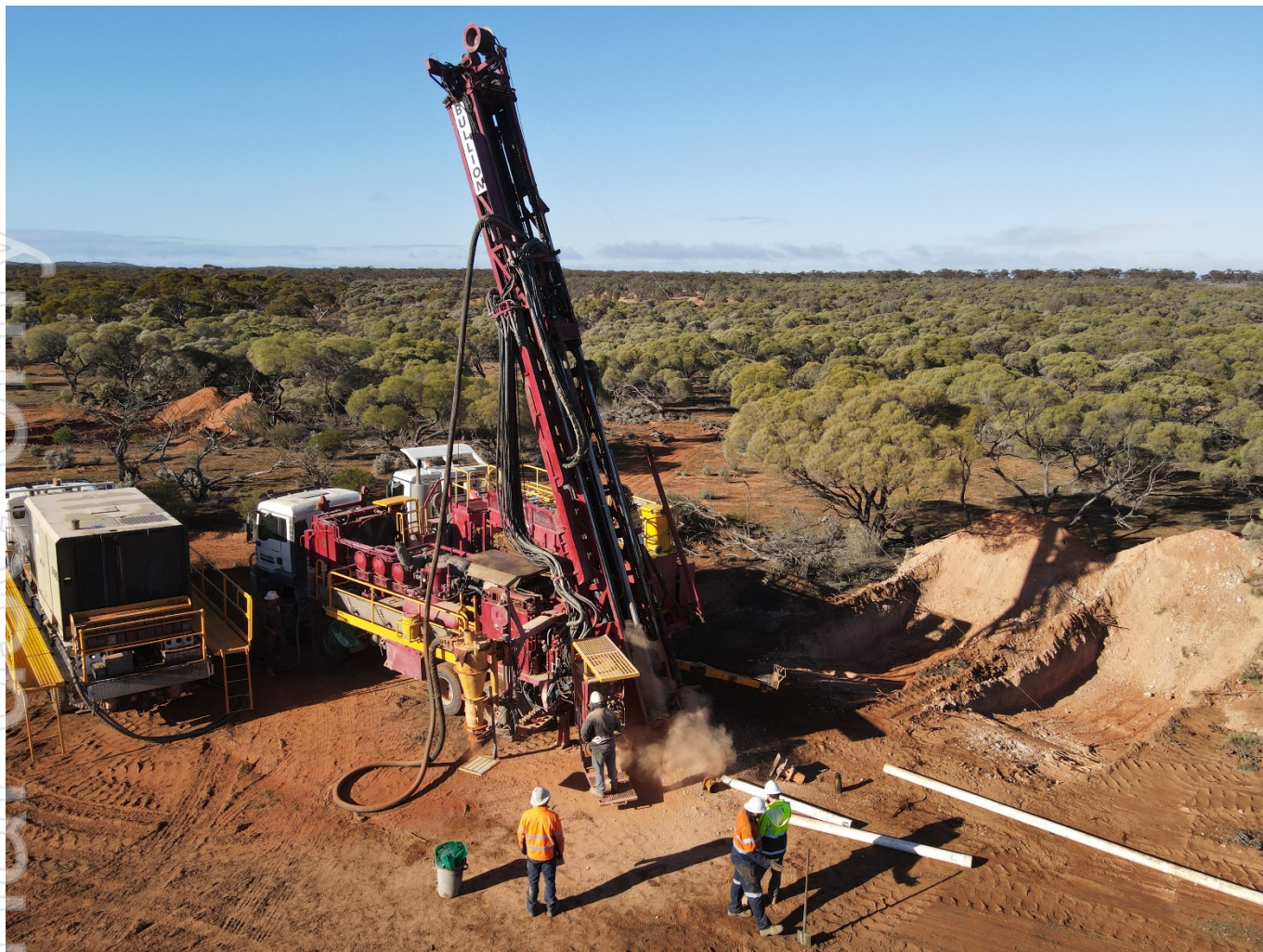
Figure 3: Picture of drill rig at the start of the program. The white PVC piping is being installed at the top - or “collar” - of the hole to stabilise the hole and allow unhindered drilling through the unconsolidated soil.
