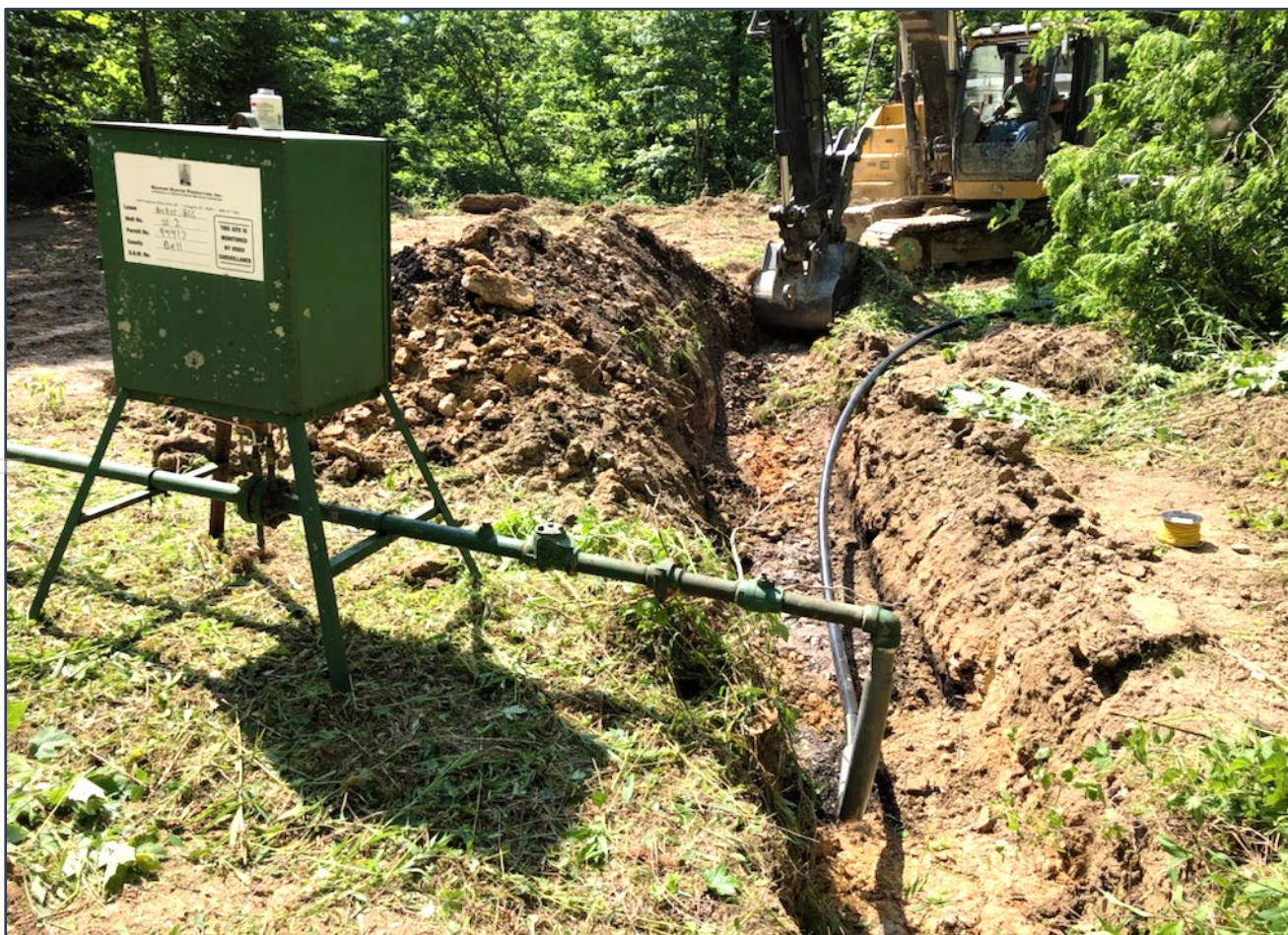
FIGURE 2: PREVIOUSLY OFFLINE GAS WELL BEING TIED BACK INTO NEWLY LAID PIPELINE
