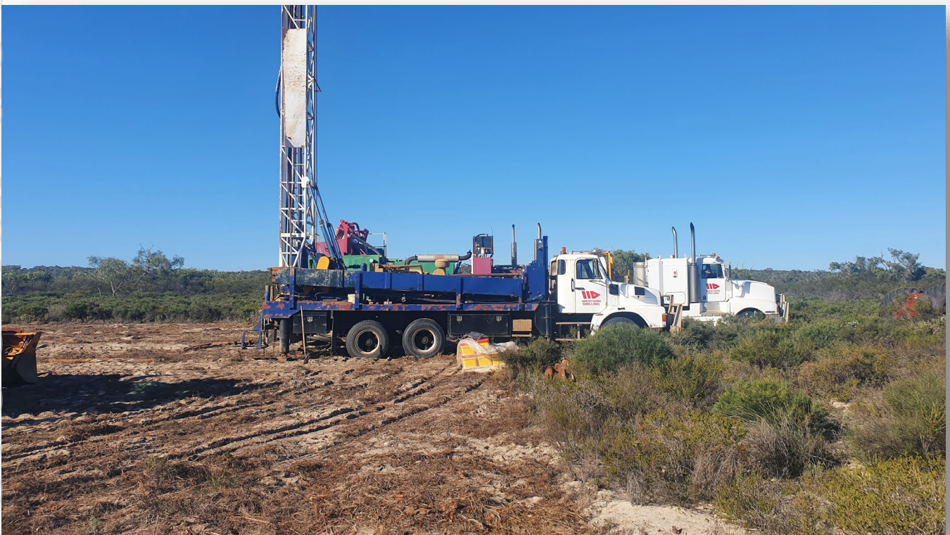
Figure 2: Water Bore Rig onsite
