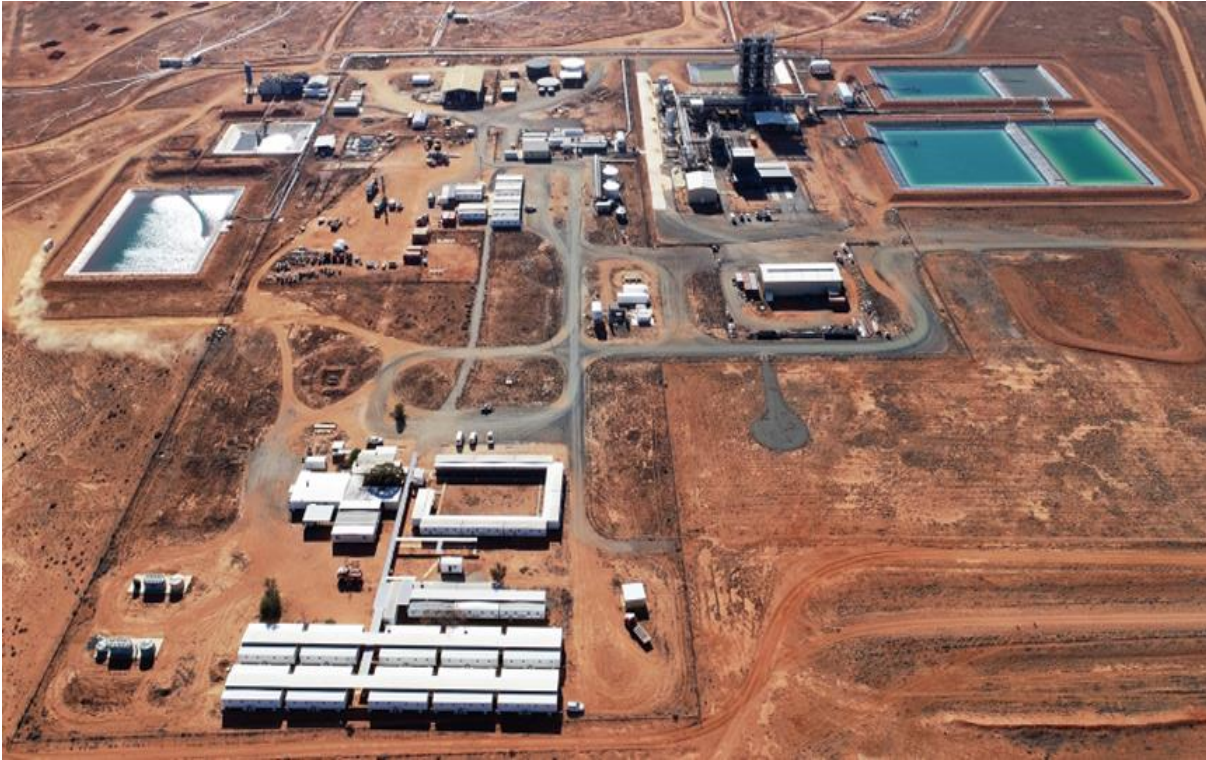
Figure 6: Existing Honeymoon process plant and infrastructure
