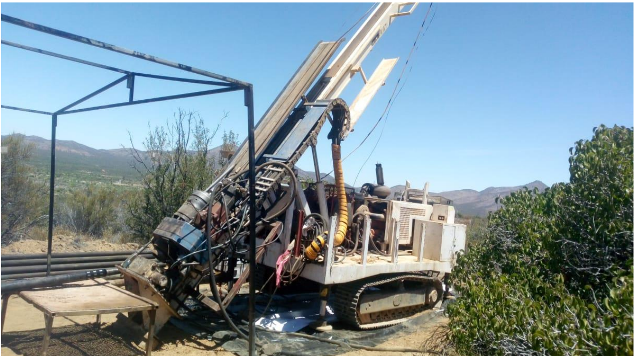
Picture 1: Track mounted drill rig positioned ready to commence drilling
