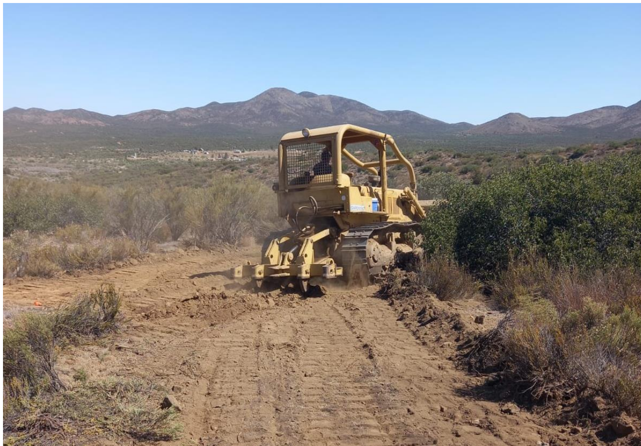
Picture 2: Dozer clearing access tracks and drill pads for drilling
